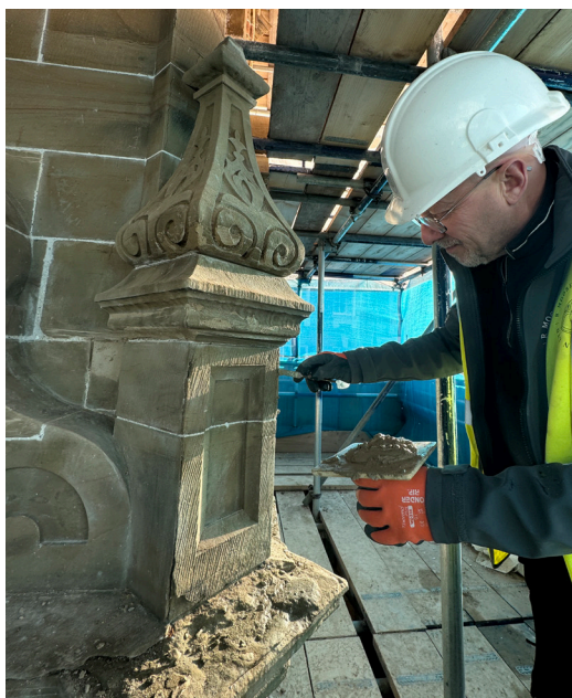
Gwaith trwsio gyda mortar calch newydd Repairs undertaken with new lime mortar
