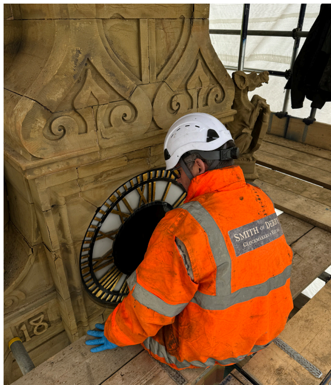
Tynnu wyneb y cloc ymaith gan y gwneuthurwyr clociau arbenigol, Smith of Derby Removal of the Clock face by specialist clock makers Smith of Derby
