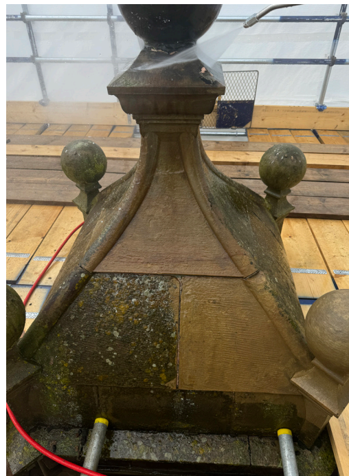
Cynnal treialon glanhau ar y gromen Cleaning trials carried out on the dome top
