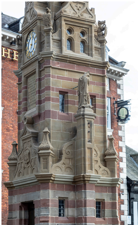
Defnyddio bandiau calchfaen a thywodfaen gwahanol liwiau (R Moore Building Conservation Ltd) Use of bands of limestone and different coloured sandstones (R Moore Building Conservation Ltd)
